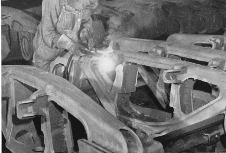
Welding surface imperfection on brake-hanger of truck side frame.
