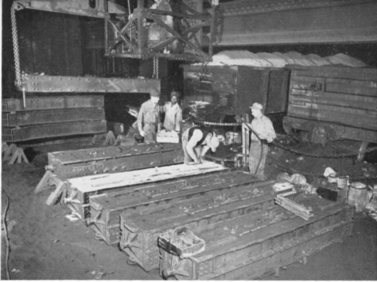
Truck bolster drags after setting cores. A cope may be seen suspended from the crane preparatory to closing and clamping to complete the mold.
