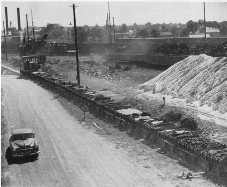
Loaded heat cars enroute to the Open Hearth Platform.
