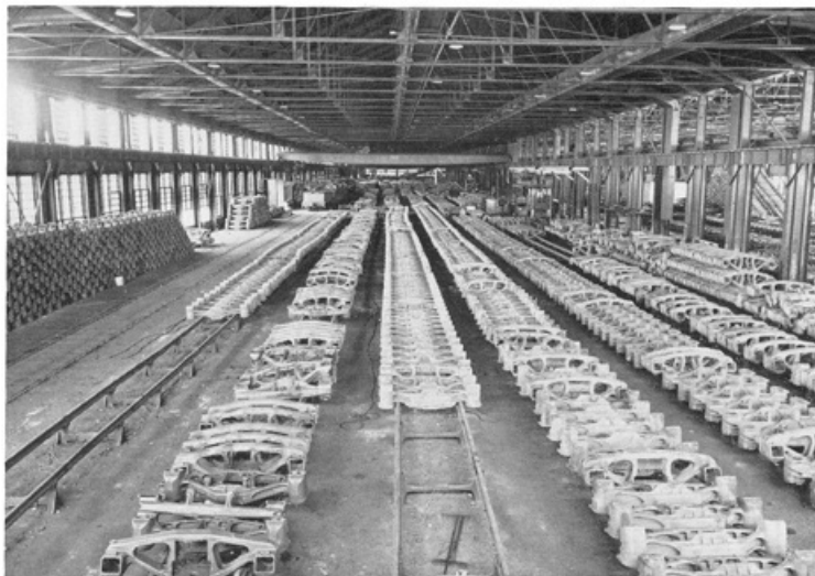
Looking north in the Frame Finishing Building. This is directly connected to the Foundry at the far end, and is 1250 feet long. Truck side frames in the foreground are ready for final inspection and gaging.
