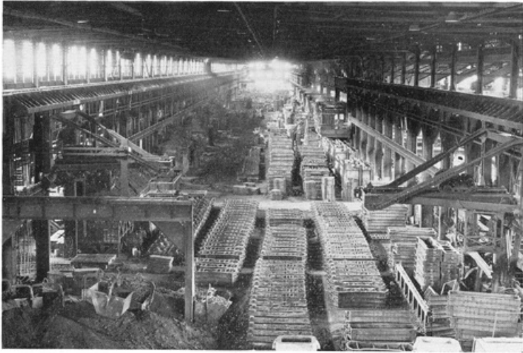
Looking west in the Pouring Bay of the Foundry. This building is 1500 feet long and is serviced by thirteen overhead cranes which range up to 60 tons lifting capacity.
