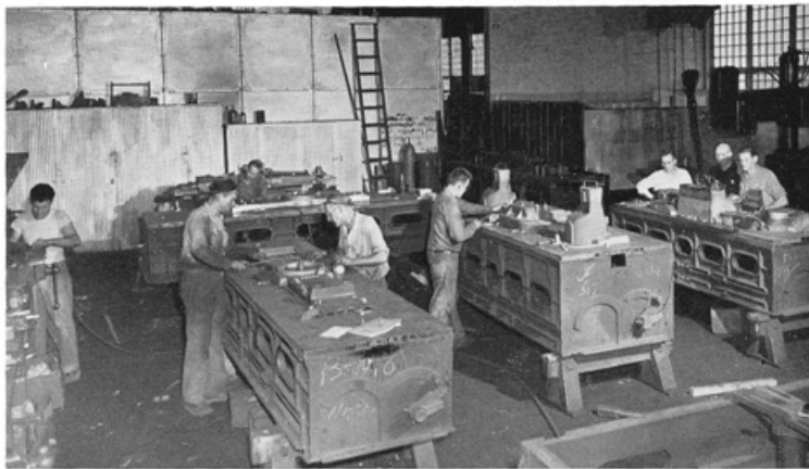
In this area of the Pattern Shop, patterns are mounted on molding machines prior to transfer to the Foundry.
