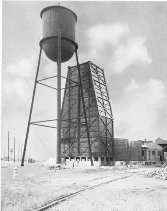
Water Softening Plant. In an average year BUCKEYE uses around 150,000,000 gallons of water, drawn from its own wells. Over two-thirds of this water is softened and otherwise treated in the facilities pictured here.
