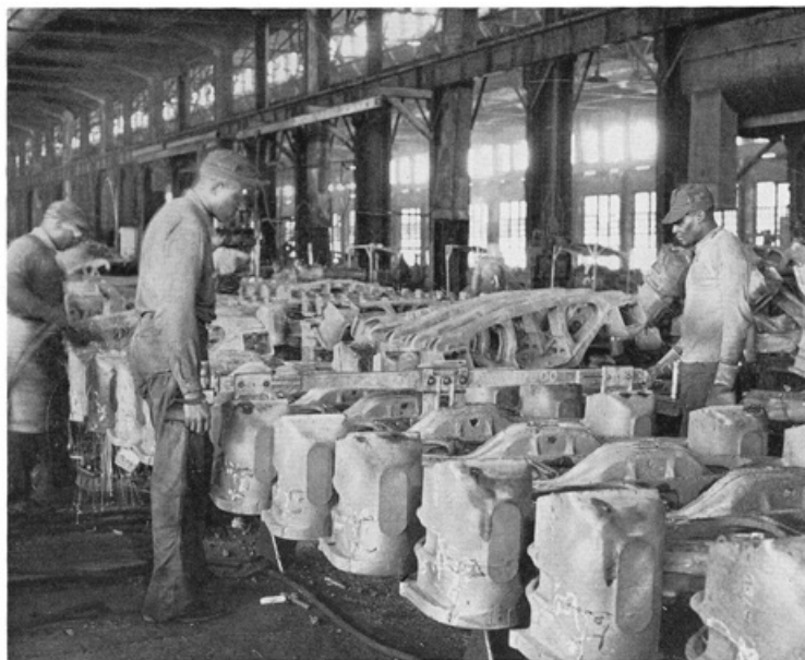
Gaging Side Frame to meet strict dimensional specifications and insure proper alignment when the frame becomes a part of a freight car truck.
